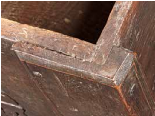
37, detail of the L-shaped stiles
